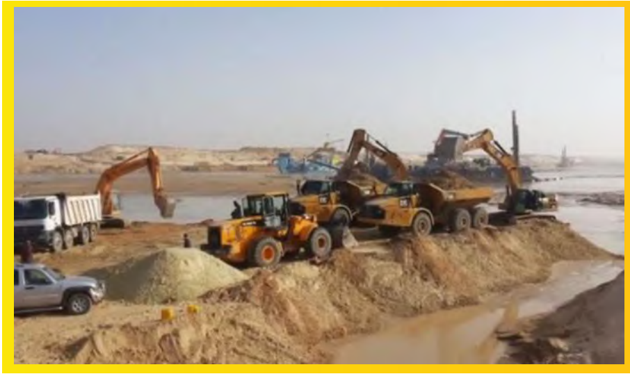
Dredging New Suez Canal
