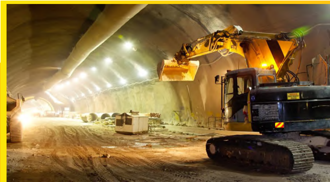
Diaphragm Walls Port said tunnels
