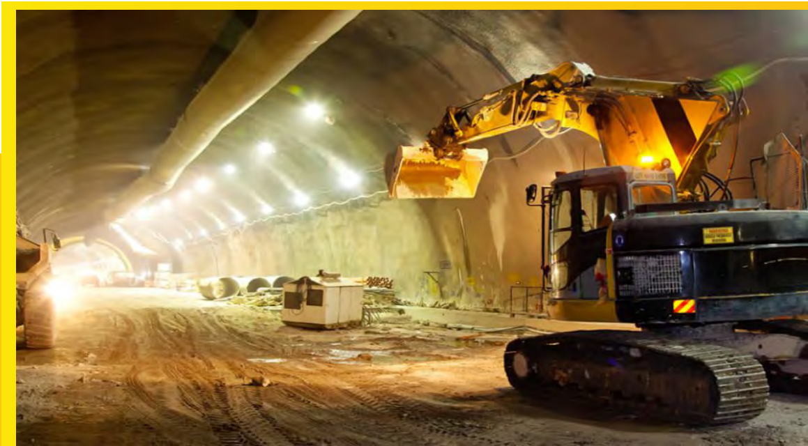
Diaphragm Walls Port said tunnels
