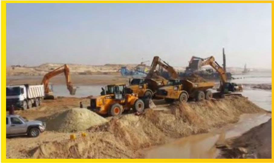
Dredging new suez canal
